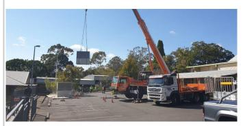
**Improvements around the parish—Air Conditioning at St Gerard's** is under construction, with the new gas powered condensers being lifted into place by crane this week. Repairs to the guttering and eaves at the back of St Gerard's will also be undertaken as part of the air conditioning installation
